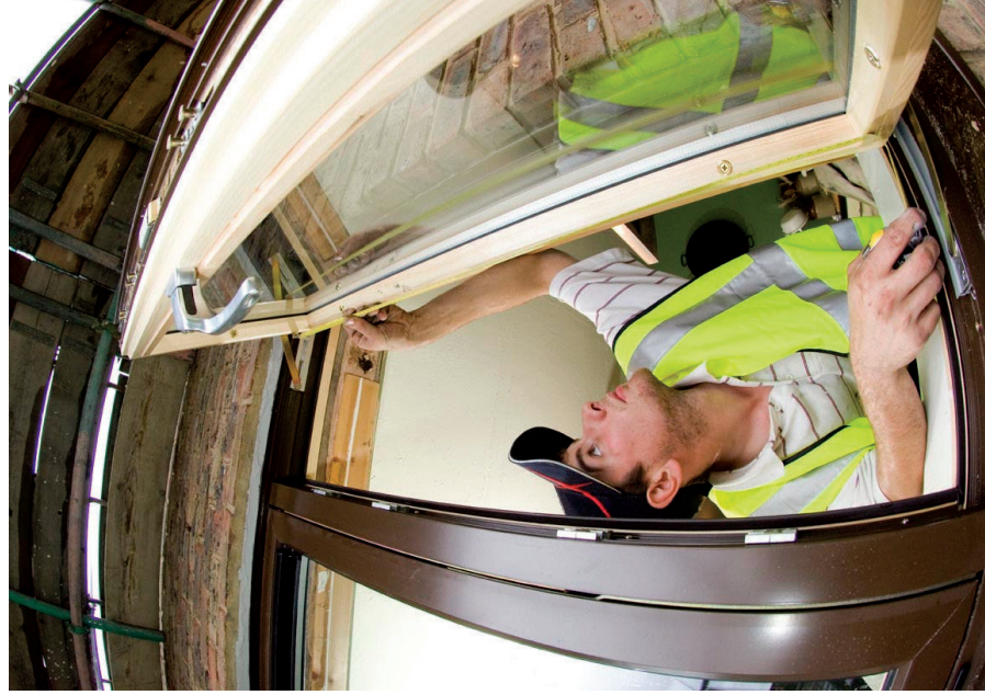
Repairs getting underway
